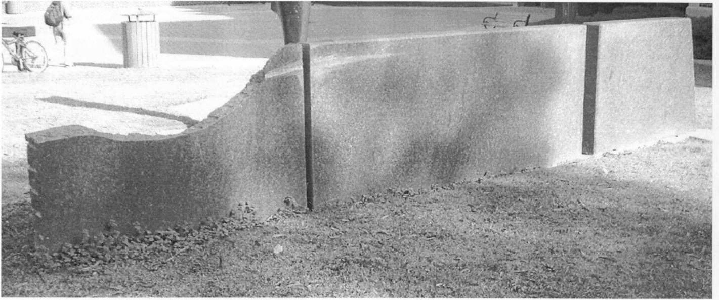
South No New signs of damage
