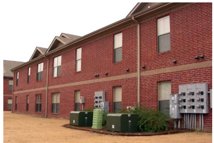
Campus utilities vary greatly in their ability to accommodate additional development.
