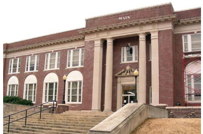
Old Main (1917) is UCA's oldest building and an illustration of the campus's Georgian architecture.
